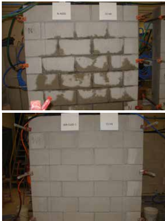
Masonry with integral water repellent mortar after 72 hours.
