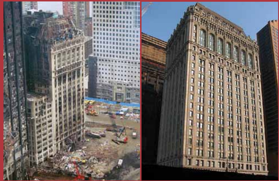
Demonstrating the resilience of CMU, the West Street Building by Cass Gilbert was reopened in 2005 after being damaged by the World Trade Center collapse and a five-day fire in 2001.
