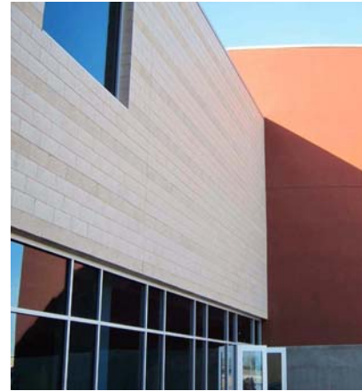
Visual interest was added to the insulated masonry walls by alternating the same hue of Mesastone and Trendstone to create a textural pattern.
