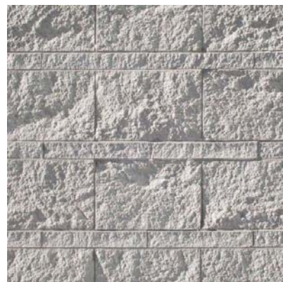
Close-up of Franklin Stone exterior wall.
