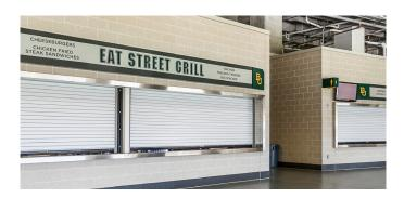
exterior wainscot along with custom colored mortar designed specifically for the job. The mortar for the entire project, including the interior and exterior brick, was supplied by Amerimix. Quality Brick Works from Robinson, Texas performed the installation.
