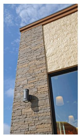
In addition to the block, Echelon supplied the Hillcrest<sup>™</sup> Stone Thin Veneer as well as the mortar, wire and damp proofing. Rather than a smooth CMU, Echelon offered SONIC a block with a unique, course texture that gives the building additional aesthetic character. Ultimately, this SONIC franchise will operate out of a sustainable and very low-maintenance
