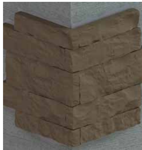
Figure 5. Stone Veneer pieces installed in a corner using a woven pattern (by switching overlapping from one side of the corner to the other)
