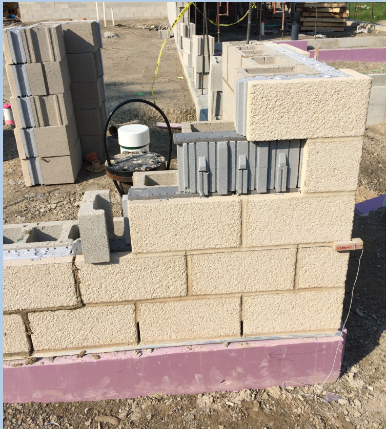
Architects on the makeover of the Banta Bowl Sports Complex in Wisconsin opted to use the ICMS for speed of construction on a limited budget.
