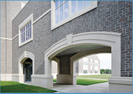
Masonry veneer was chosen for its look of natural stone without the high cost.
