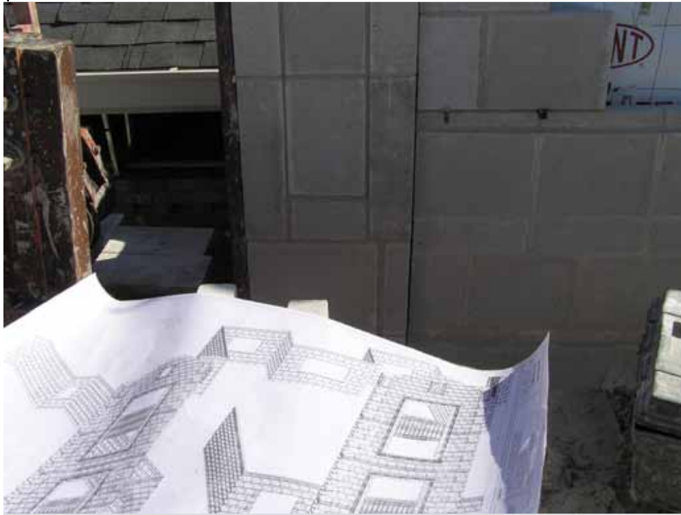
Modeling can help streamline the staging of a masonry job.
