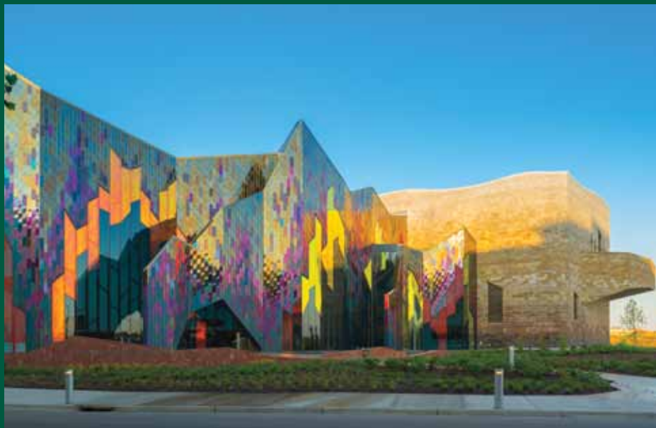
The forward-looking Prairiefire Museum incorporates full-depth stone veneer and a front balcony faced with a 1-inch thin veneer.
